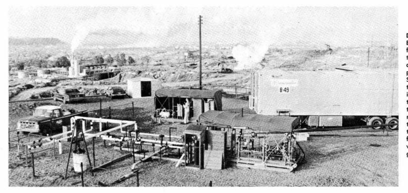
**DEEP STEAM test site near** Bakersfield, Calif. — In foreground is the skid containing the steam generating unit and associated pressure and flow gages. Skid in background contains test controls and instrumentation. At left is the plumbing leading to the injection well and, at right, a Sandia instrumentation trailer. Plumes in the background are vapor from scrubbers on conventional surface steam
